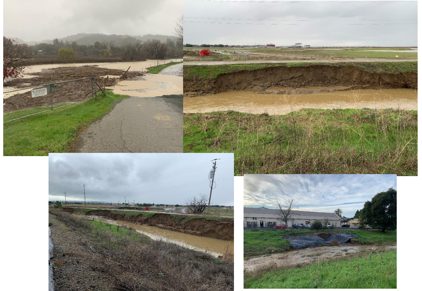
Facilities during recent 2022 storms
