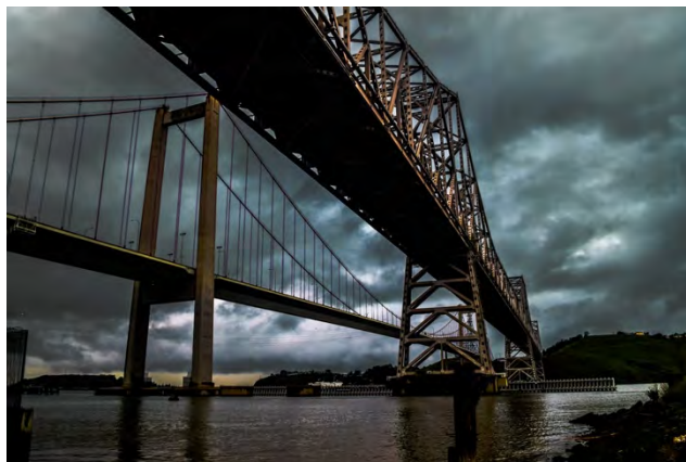
Photo of the Carquinez Bridge by Antonio Tamayo, a Richmond-based photographer interviewed in this study. [Image description: Two metal bridges above a bay are seen from the perspective of someone standing below them. Behind the bridges the sky is an ominous cloudy grey, with a bit of light shining through.]
