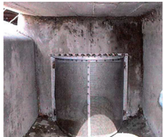
Inside of a drainage inlet retrofitted with a trash capture device.
