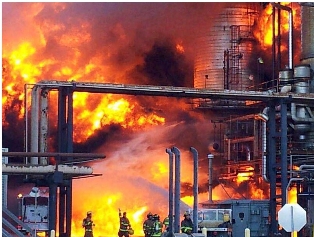
Chevron Richmond Refinery, 6 Aug 2012. Image: CSB
