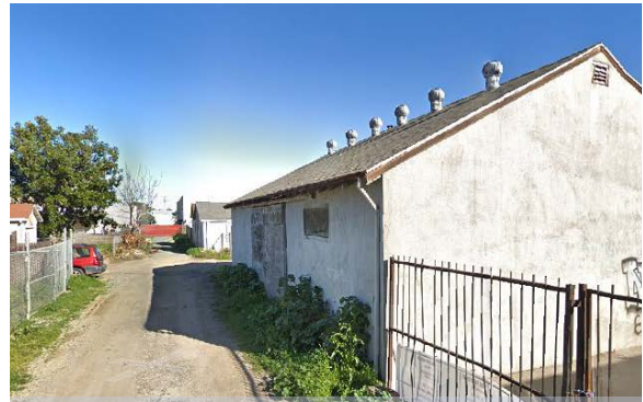
362 Parker Ave _ Office
