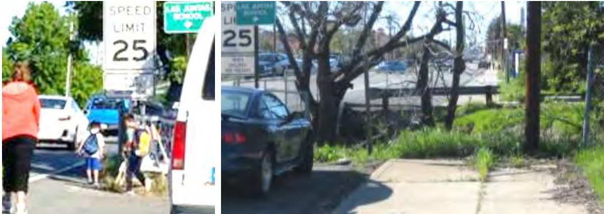
Figure 6: Without a continuous path, pedestrians walked in the roadway shoulder
