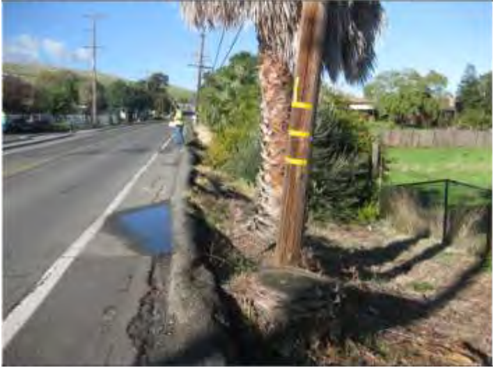
Figure 8: Pre-Construction Image of Pacific Avenue (above)
