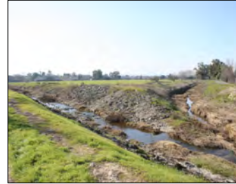
Looking upstream at Sand Creek confluence
