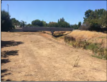
Looking upstream to Central Ave. Bridge
