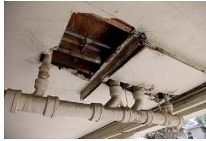
The simple wood construction and open holes in this carport ceiling, shown during an April inspection of an Oakland apartment building, would not prevent a vehicle fire from threatening residents above.
