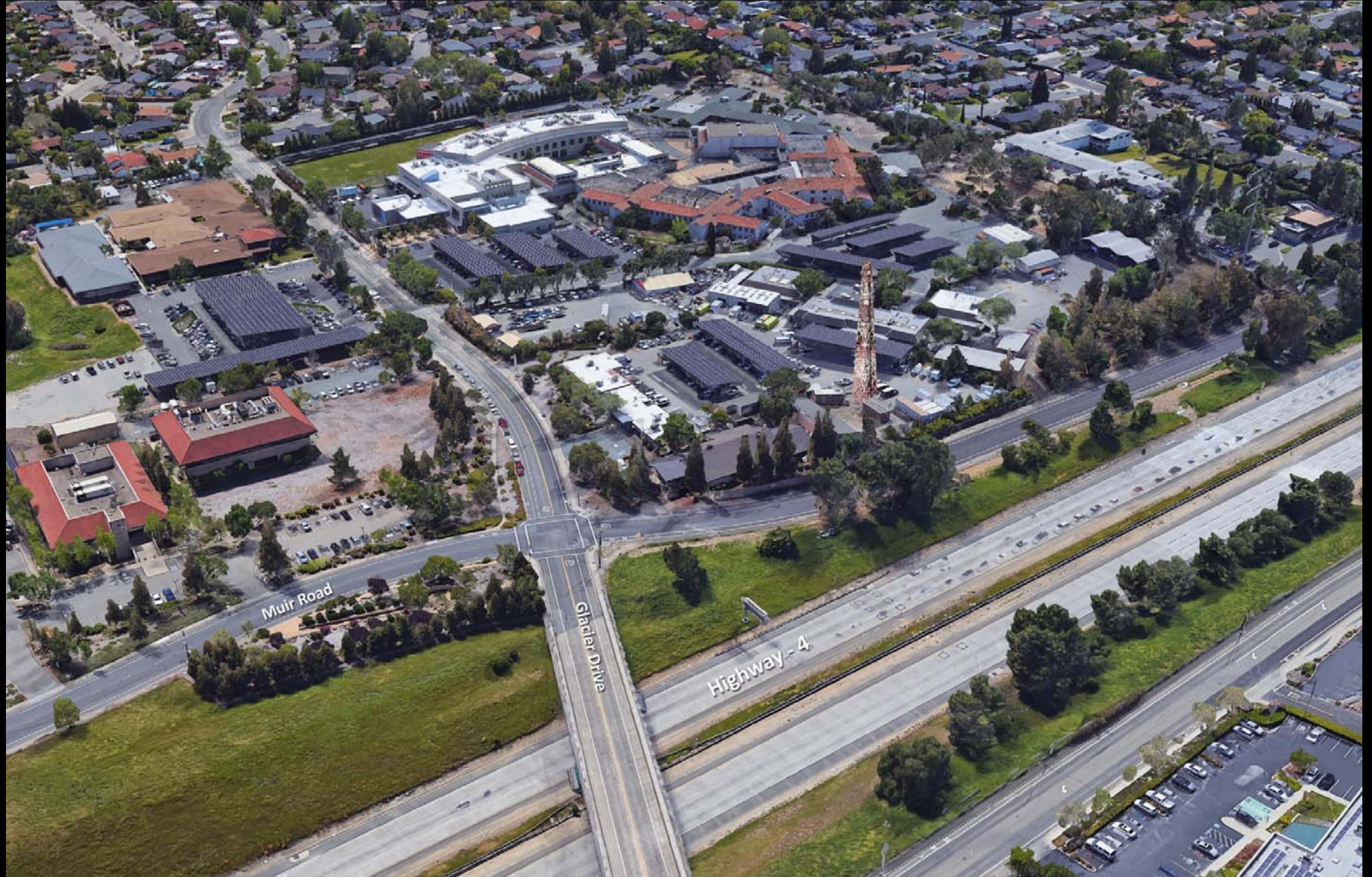
CAMPUS AERIAL PHOTO
