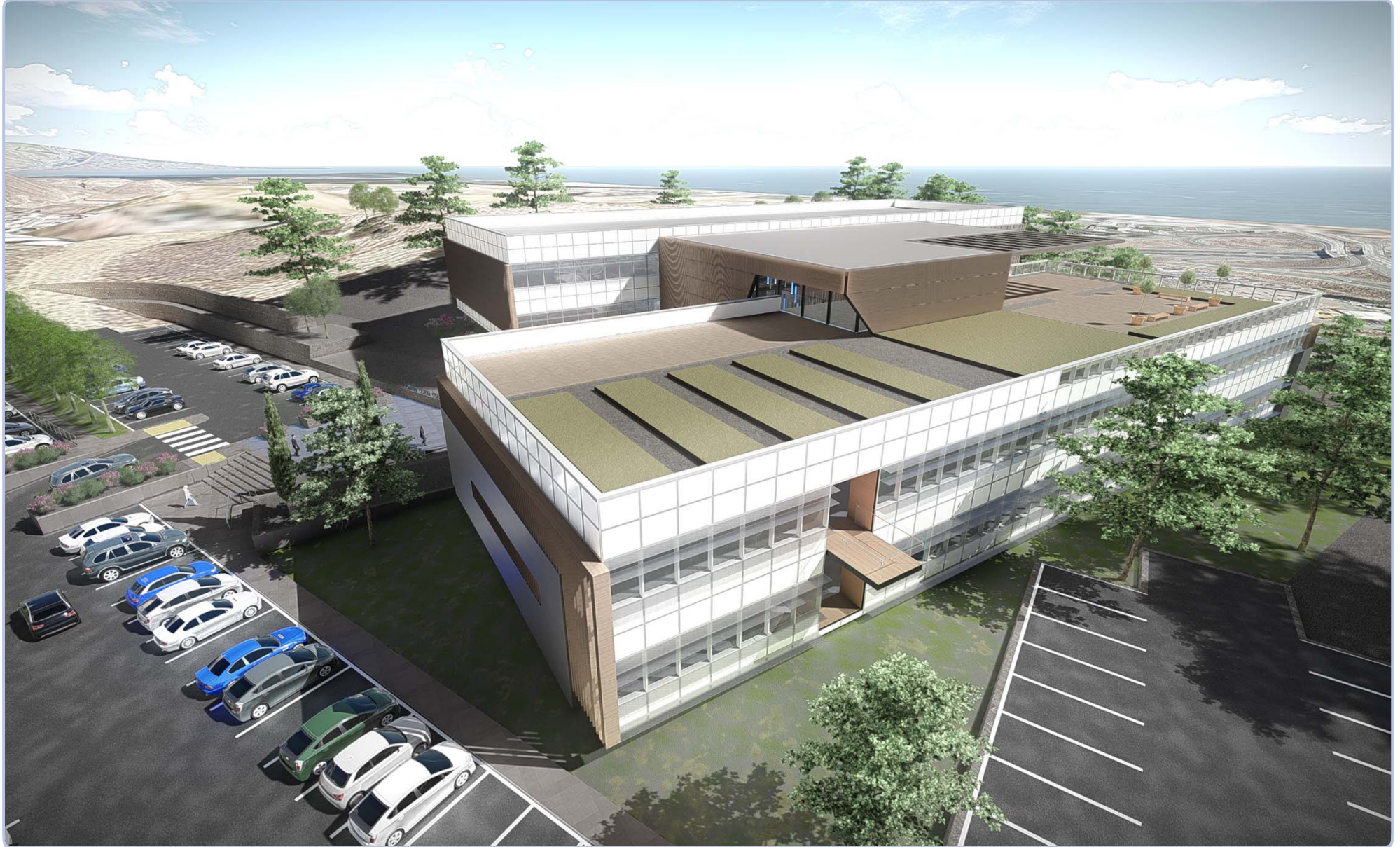
AERIAL VIEW LOOKING NORTH
