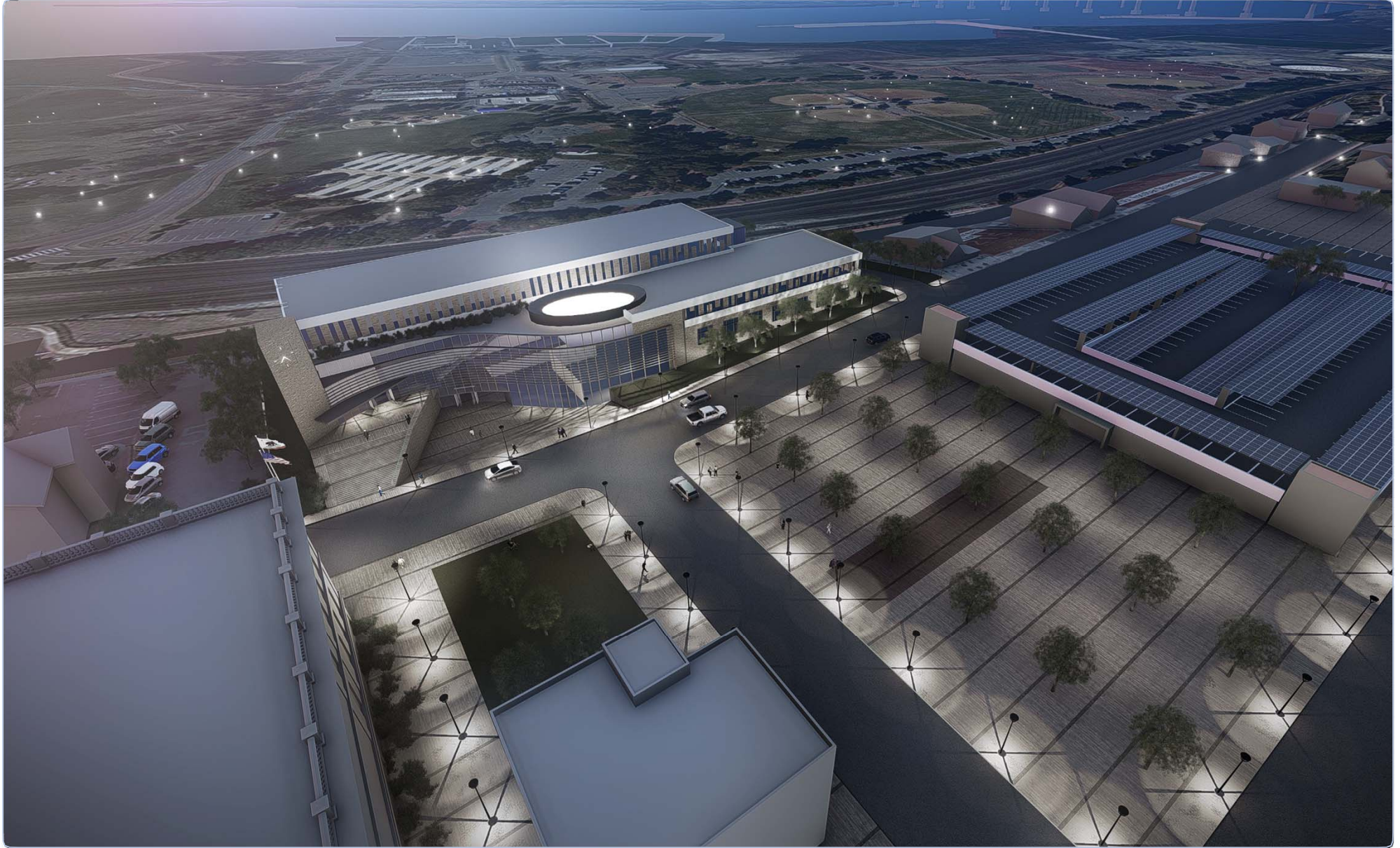
AERIAL VIEW LOOKING NORTH
