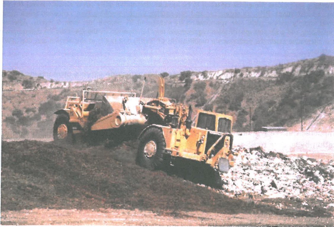
From Exhibit C – Figure 4. A scraper lays processed green waste ADC over a compacted refuse cell
