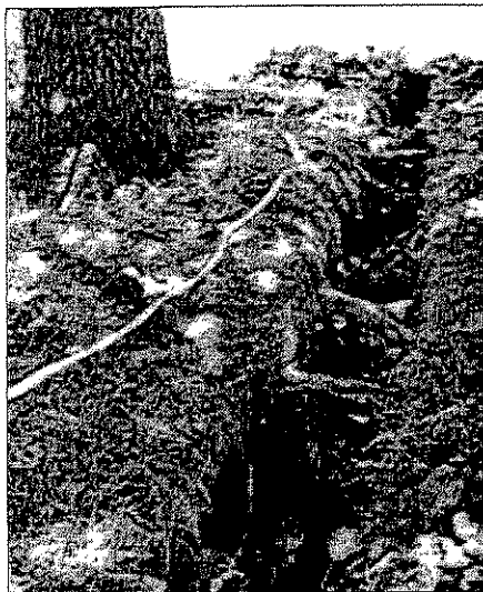
Pneumatic or hydraulic tools can be used to remove soil around tree roots to determine their number and size, to expose them so they can be cut with a saw, or to thread pipes or conduit under them rather than cutting.
