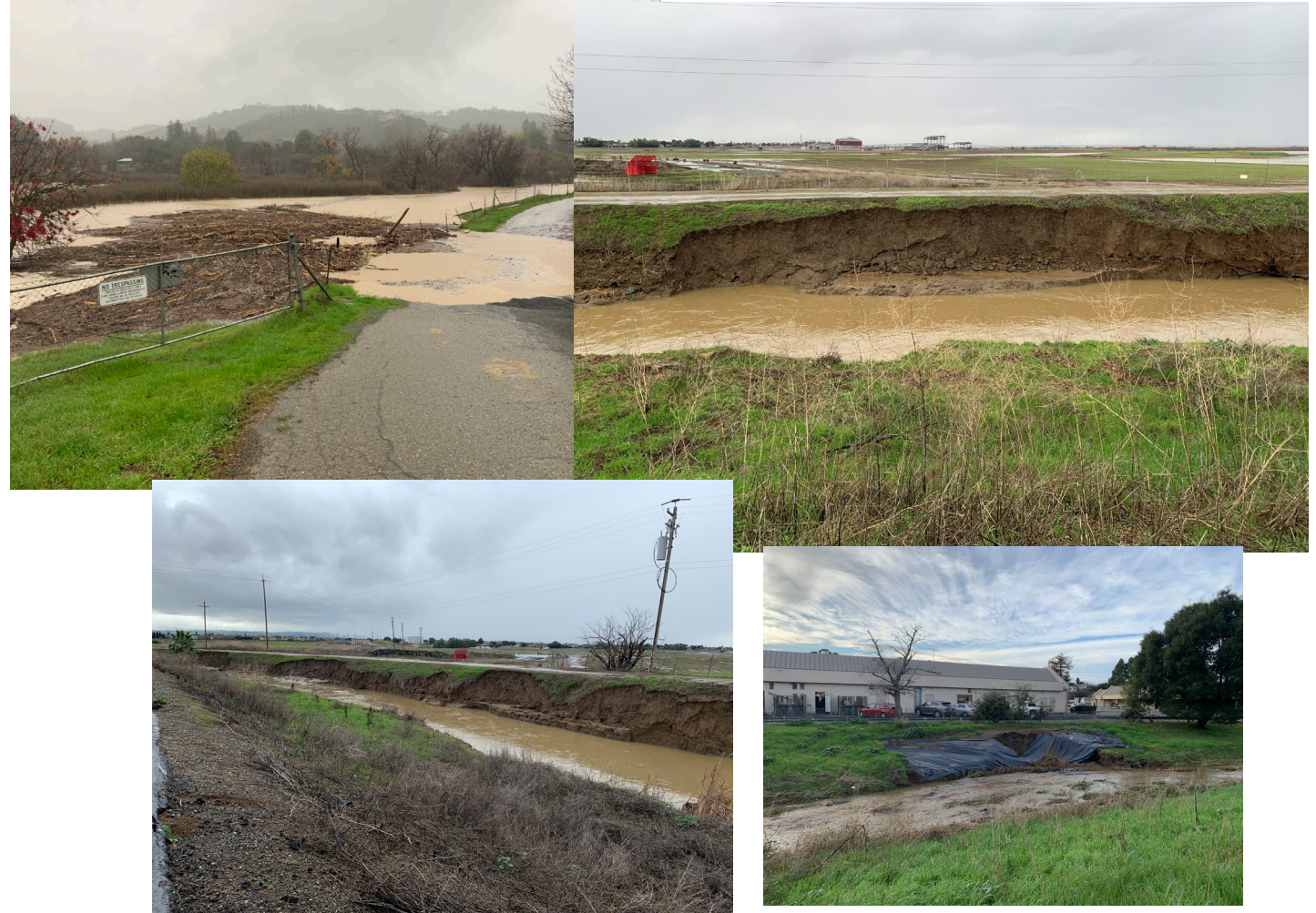
Facilities during recent 2022 storms
