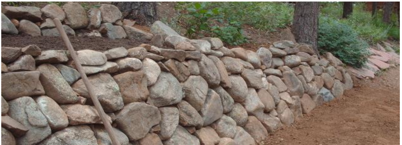
Figure 4-17. Stacked rock retaining wall
