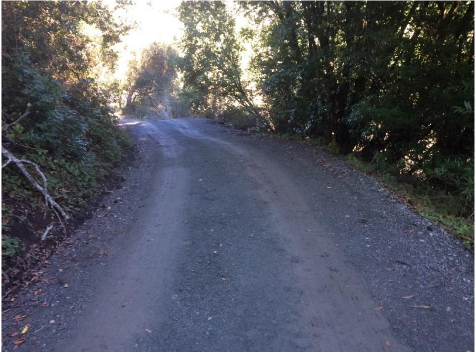
Figure 4-11. Lime-treated base rock surface
