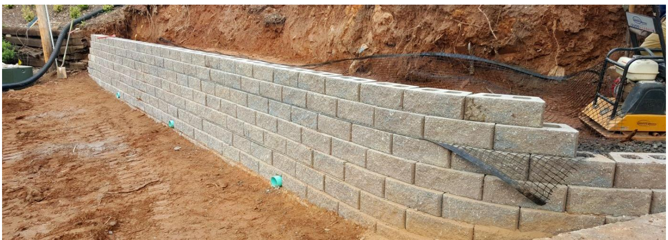
Figure 4-18. Concrete masonry unit retaining wall (could be covered with soil and planted on
