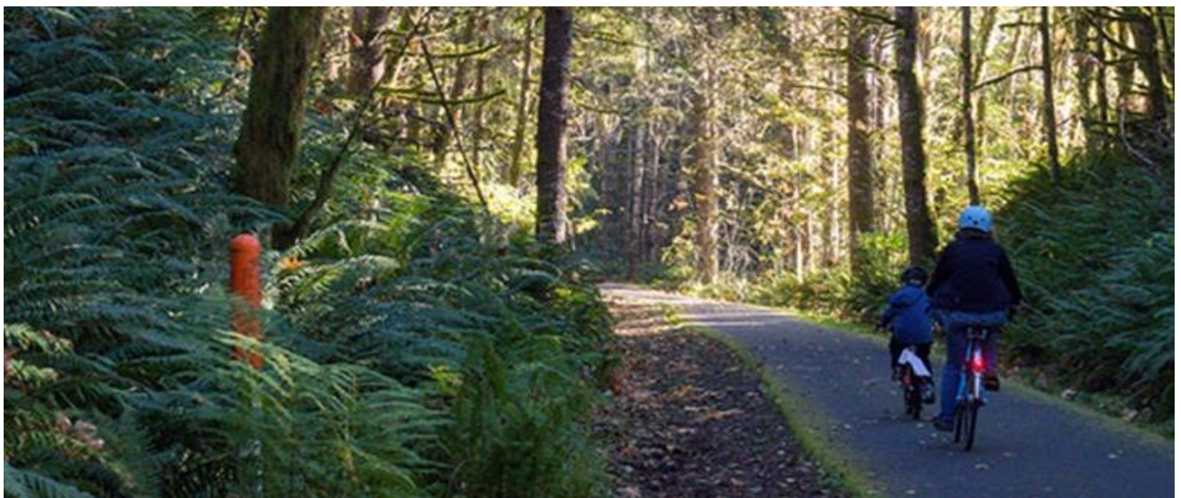
Figure 4-8. Example of an asphaltic concrete (AC) trail
