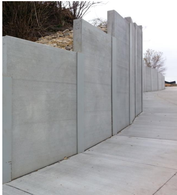
Figure 4-15. Concrete retaining wall
