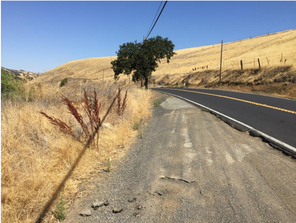
Figure 5-10. Wide unpaved shoulder with turnout
