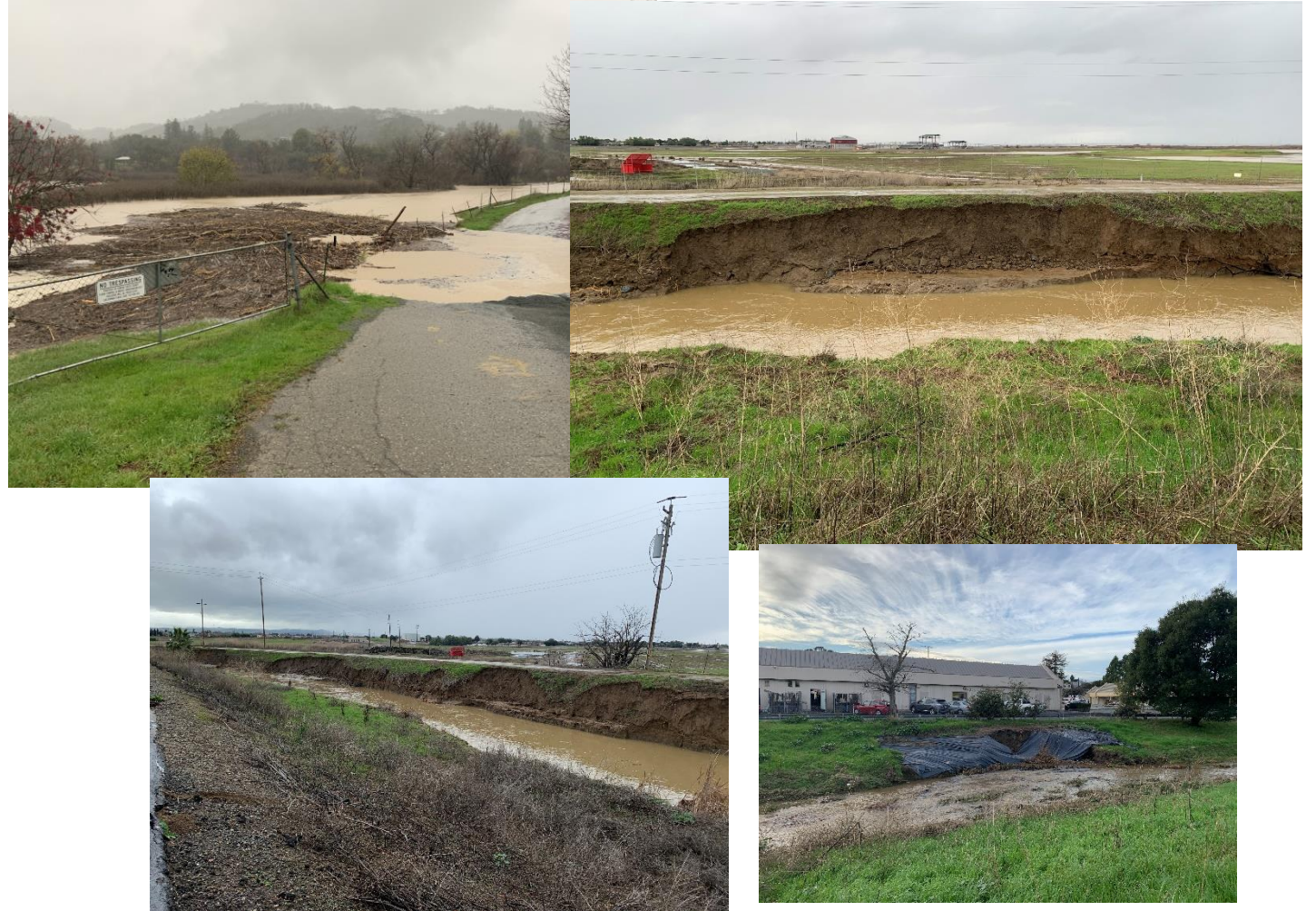
Facilities during recent 2022 storms
