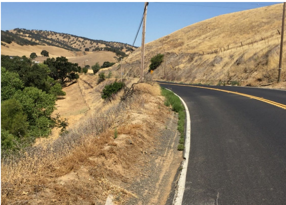
Figure 5-11. Portion with no shoulder
