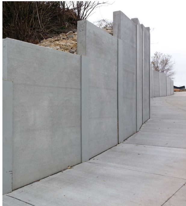
Figure 4-15. Concrete retaining wall
