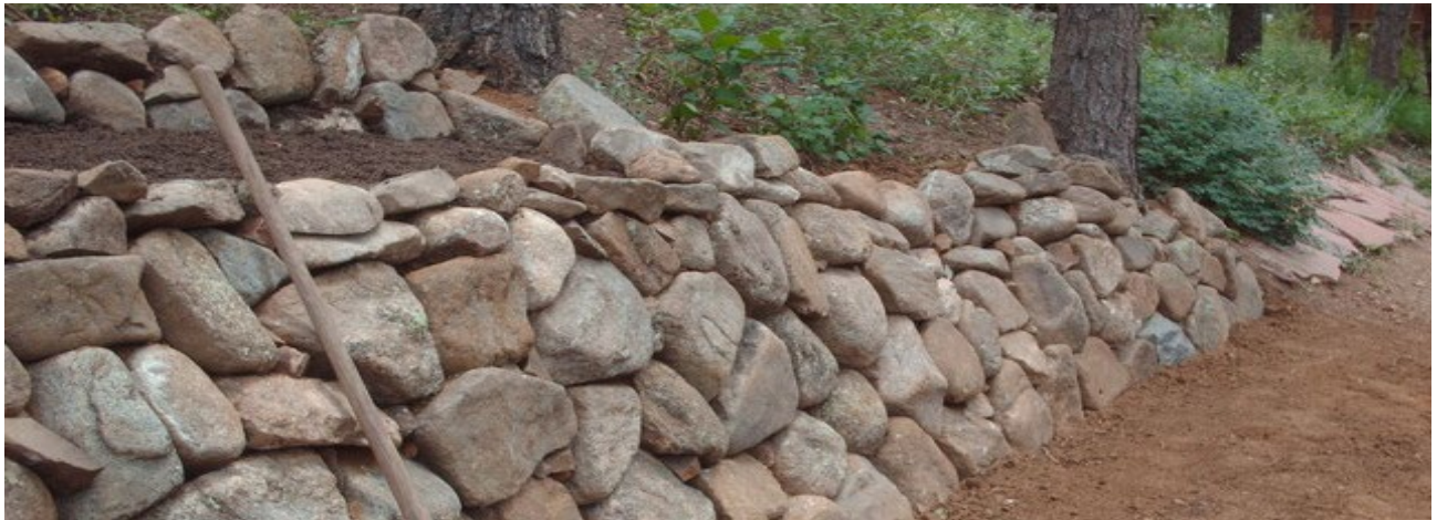
Figure 4-17. Stacked rock retaining wall
