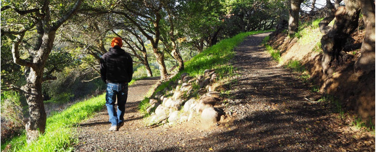
Figure 4-9. Example of base rock surfaced multi-use trail in Marin County
