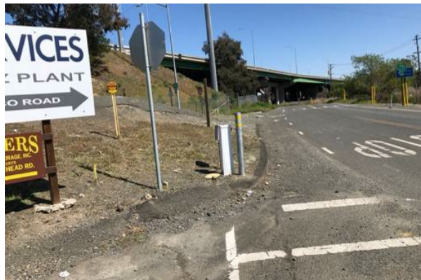
Looking east, north side of Mococo Road between Bridgehead and Trailhead. Existing bike lanes used by pedestrians as Bay Trail route. Potential route for new shared-use trail or pedestrian sidewalk with Class IV bikeway.
