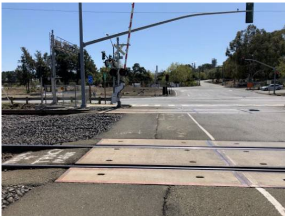
Looking south along east side of Mococo Road at existing bike lane and potential location of shared-use trail.
