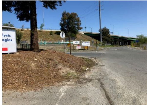
Looking east, potential location for potential new shared-use trail or pedestrian sidewalk adjacent to Mococo Road between Bridgehead Road and access driveway.
