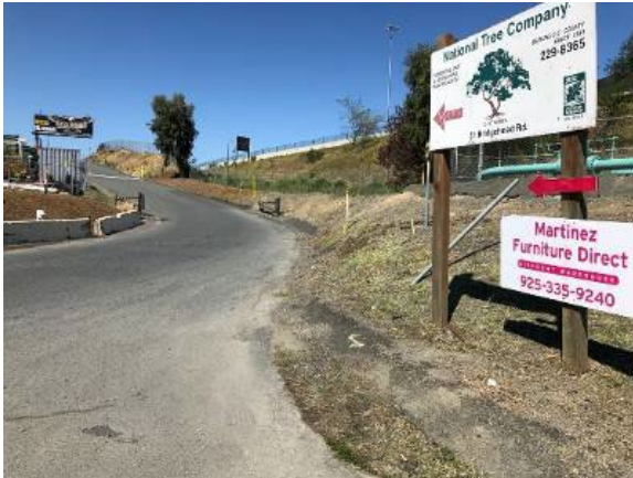
Looking north, potential new shared use trail alignment parallel to or in place of Bridgehead Road.
