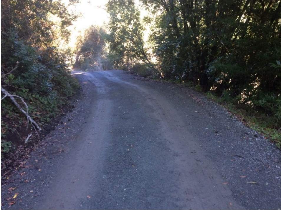
Figure 4-11. Lime-treated base rock surface
