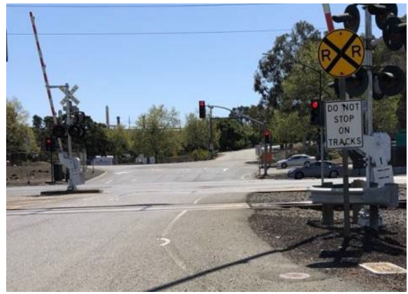
Looking south along west side of Mococo Road at existing bike lane and potential location of shared-use trail.
