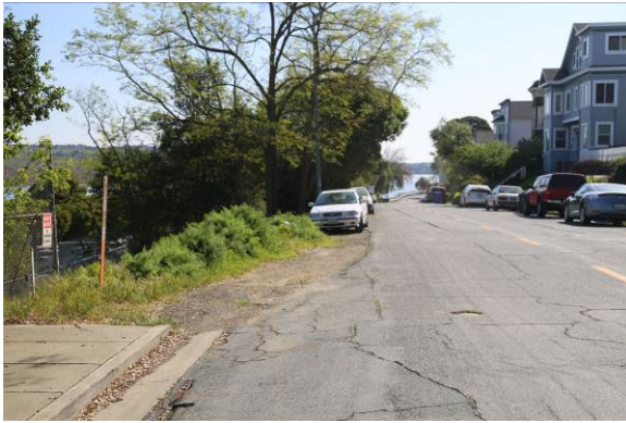
Loring Ave. east of Jackson Street
