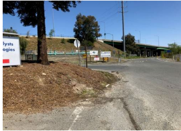
Looking east, potential location for potential new shared-use trail or pedestrian sidewalk adjacent to Mococo Road between Bridgehead Road and access driveway.
