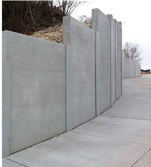
Figure 4-15. Concrete retaining wall
