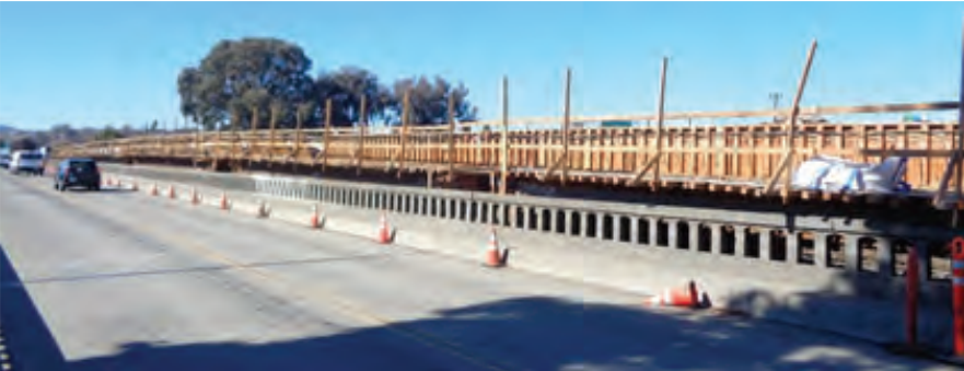
Marsh Drive Bridge Under Construction
