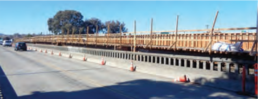
Marsh Drive Bridge Under Construction
