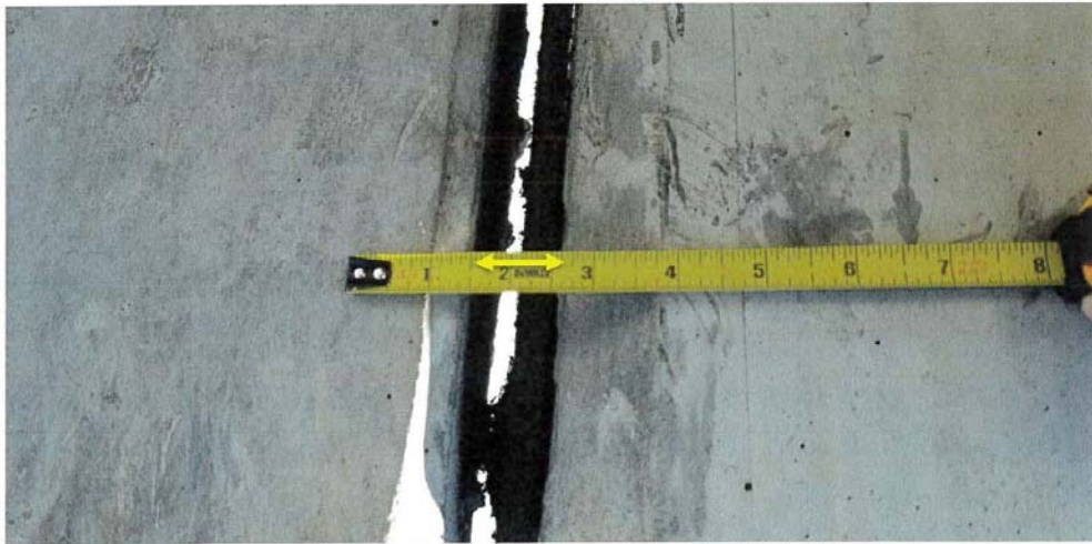
3. Separation in parapet wall measured approximately 1-1/8 inch
