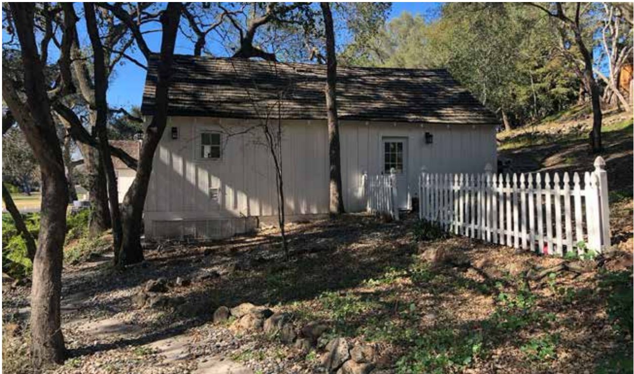
Fig.17 – 1897 Calle Arroyo – Rear of garage, looking west
