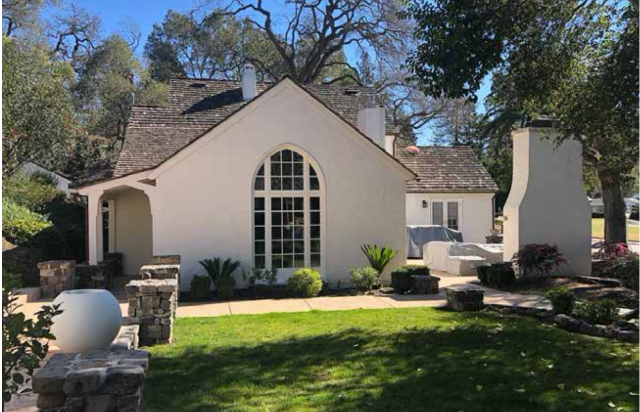
Fig.9 – 1897 Calle Arroyo – West wing, from west
