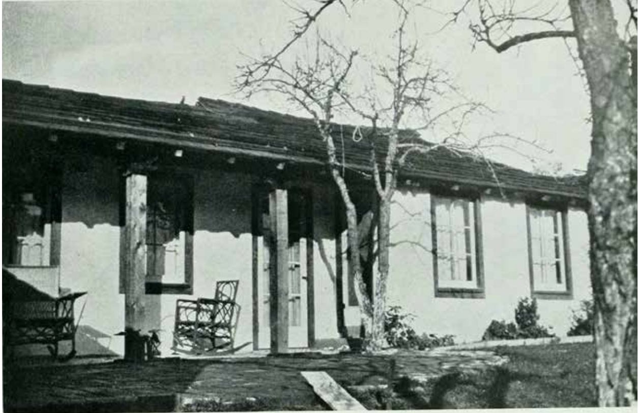
HOUSE FOR MR. AND MRS. MONROE GREENWOOD, MOUNT DIABLO, CALIFORNIA Frederick H. Reimers, Architect
