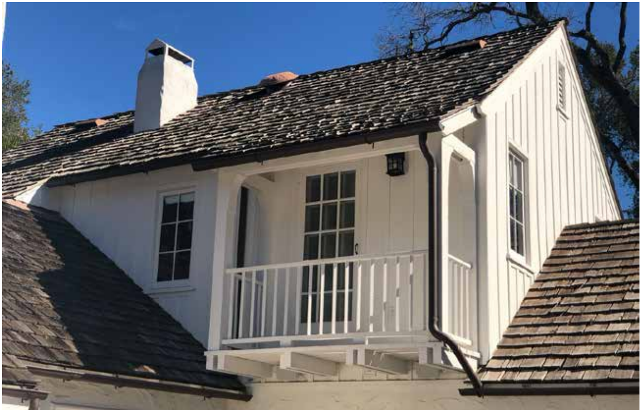
Fig.10 – 1897 Calle Arroyo – Balcony at upper west side
