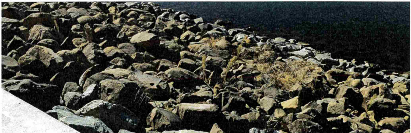
Photo 1 – Upstream rip-rap slope in satisfactory condition with mild vegetation.
