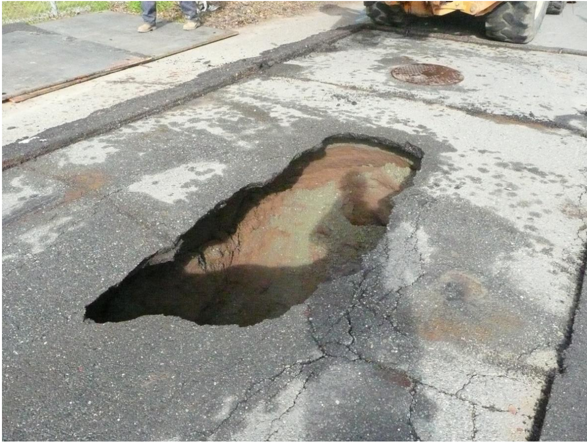
Figure 2-B. Roadway sinkhole due to storm drain pipe collapse.
