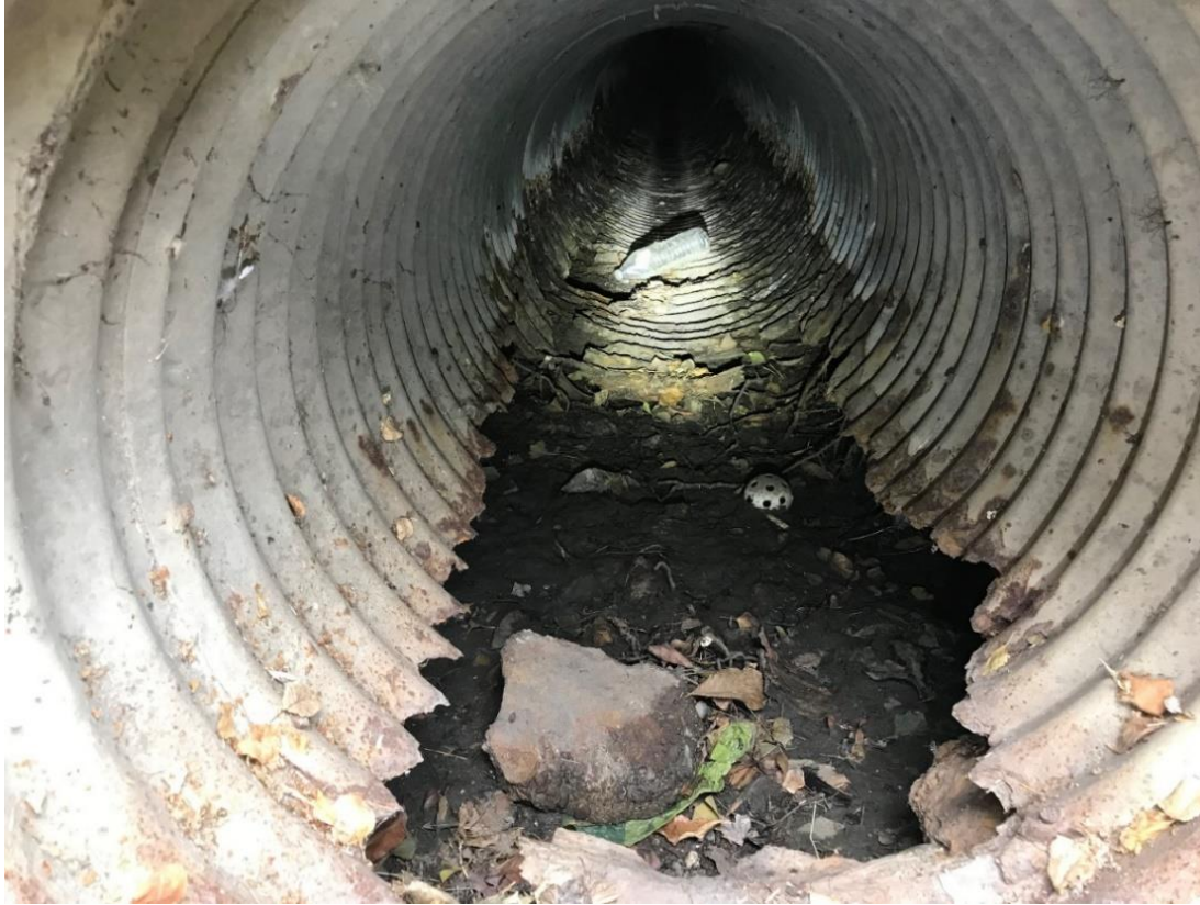
Figure 2-C. Most metal pipes throughout the County are greater than 50 years old (well exceeding their intended lifespan) and the bottom has rusted through, or will soon. This pipe is considered as failed, and may soon collapse to create a sinkhole.
