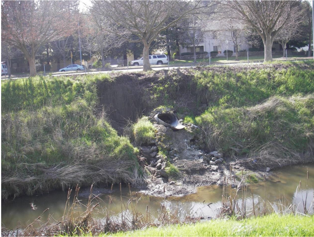
Figure 1-D. Creek bank erosion and storm drain pipe failure on Rodeo Creek.
