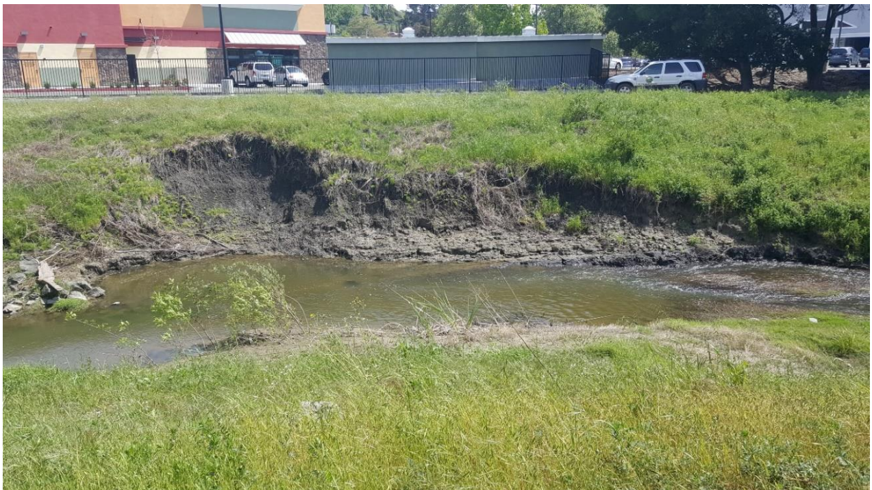
Figure 1-C. Creek bank erosion on Pinole Creek.
