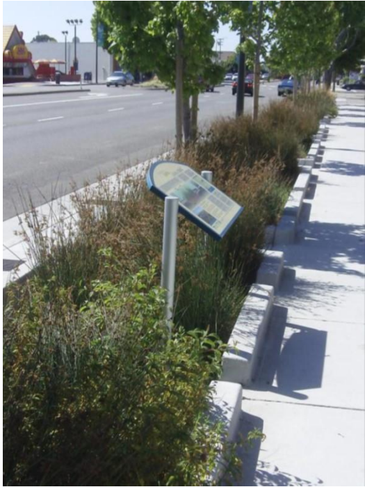
Figure 5-A. An example of green infrastructure along a street in San Pablo. It cleans runoff from streets and sidewalks, provides urban greening, and provides climate change resiliency.
