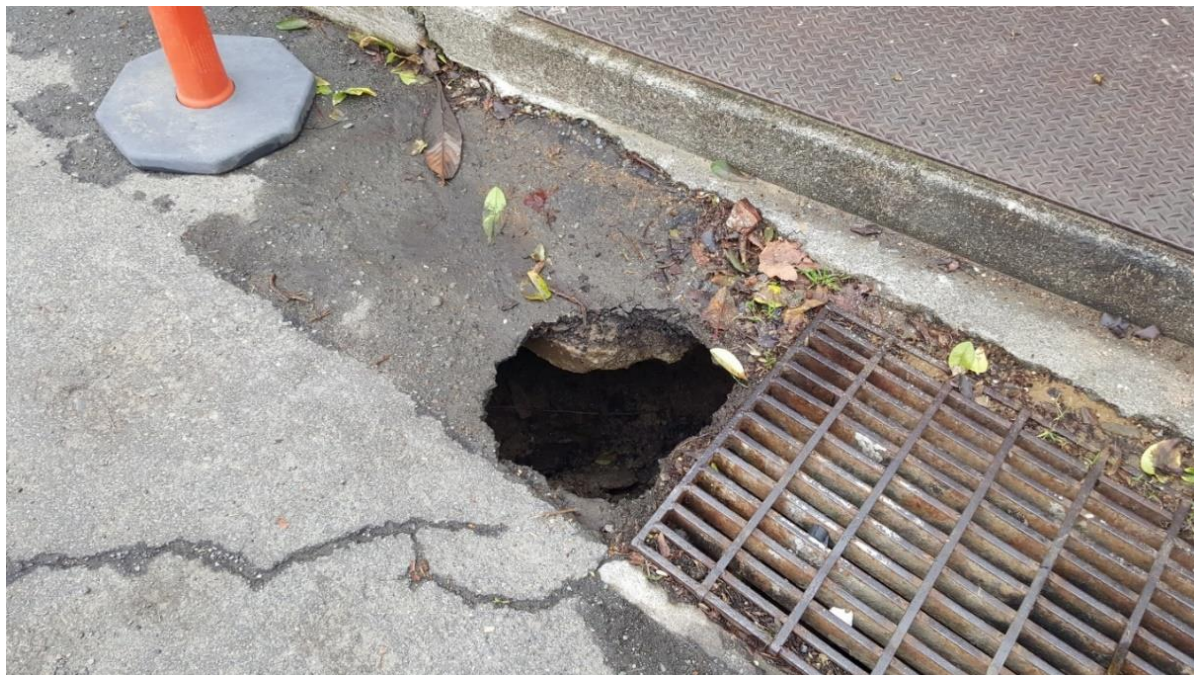
Figure 2-A. Roadway sinkhole due to storm drain pipe collapse which is a safety concern for motorists, bicyclists, and pedestrians.
