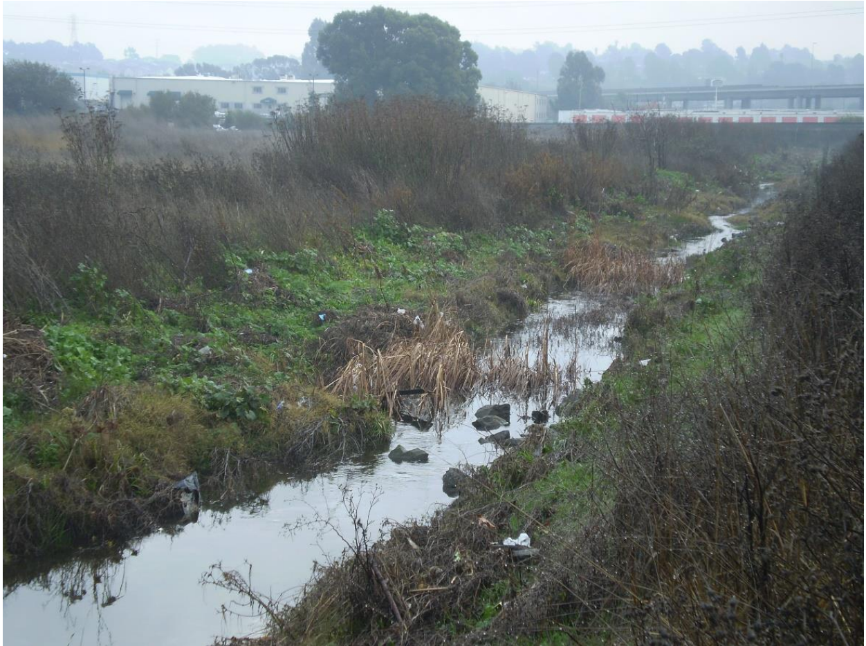
Figure 1-B. Silt build up due to lack of routine maintenance in Rheem Creek due to lack of funding.
