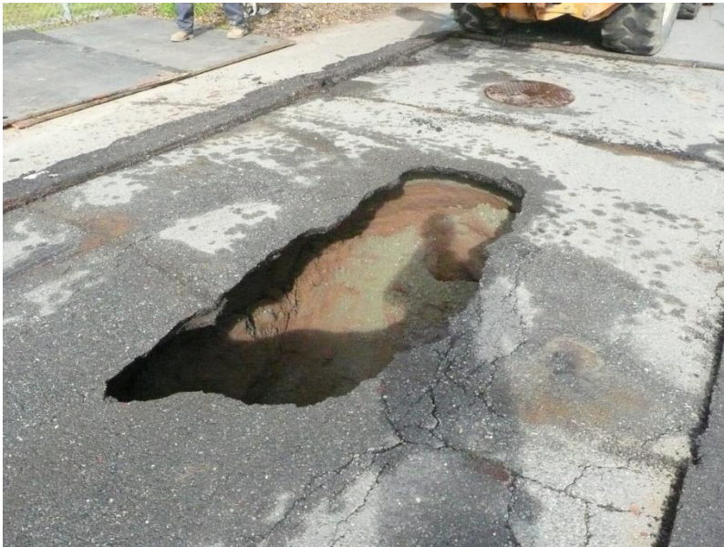
Examples of failed storm drains and resulting pavement damage
