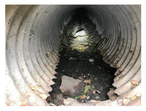
**Figure 2-C.** Most metal pipes throughout the County are greater than 50 years old (well exceeding their intended lifespan) and the bottom has rusted through, or will soon. This pipe is considered as failed, and may soon collapse to create a sinkhole.
