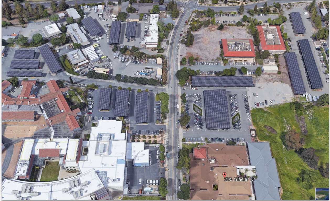
Figure 2: Contra Costa County has established itself as a leader in DER as illustrated by this Google image showing a high penetration of PV parking lot canopy systems at an important municipal complex on the corner of Muir and Glacier in Martinez.
