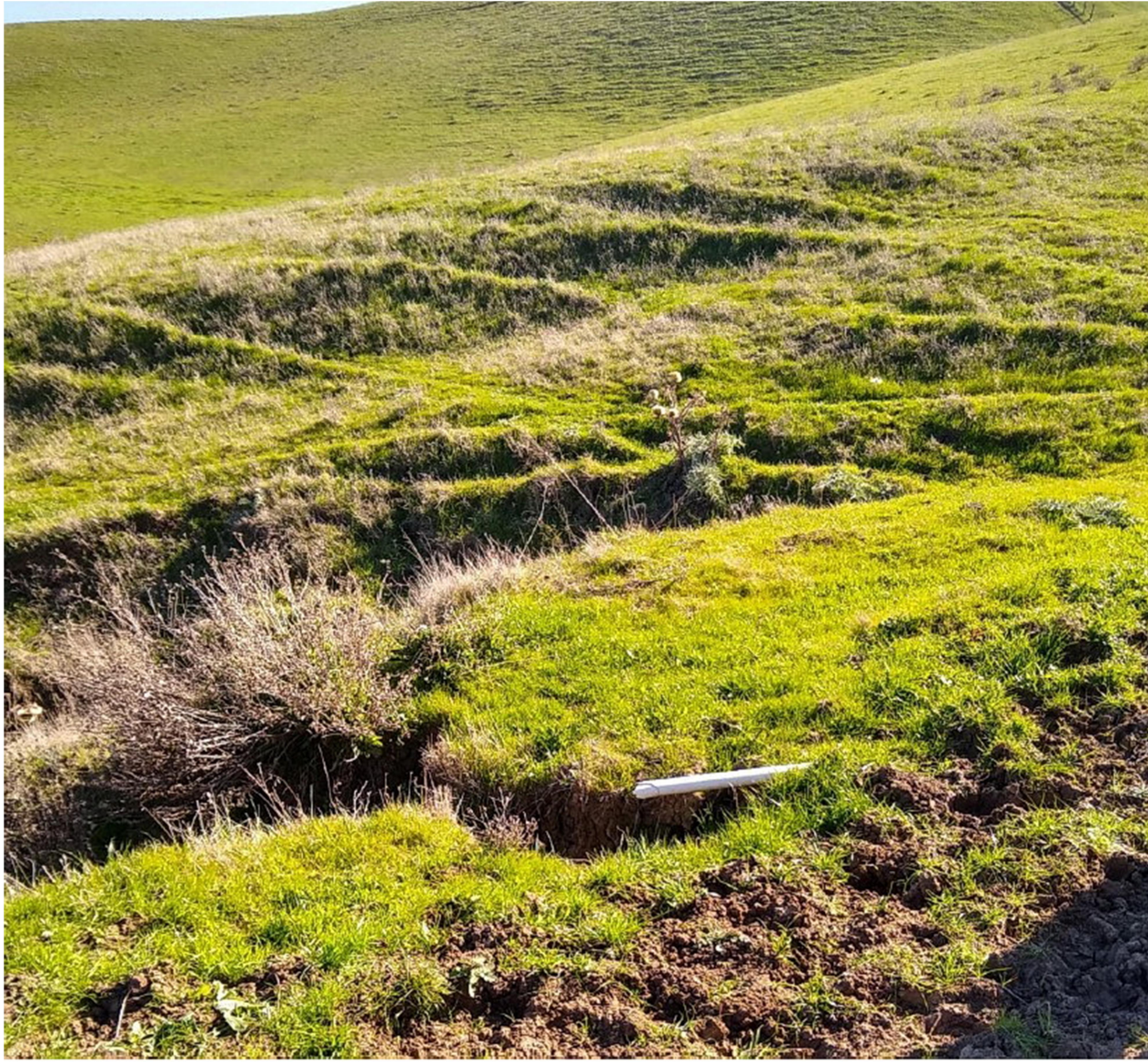
Several headcuts downstream of road crossing, near observed bedrock exposure.
