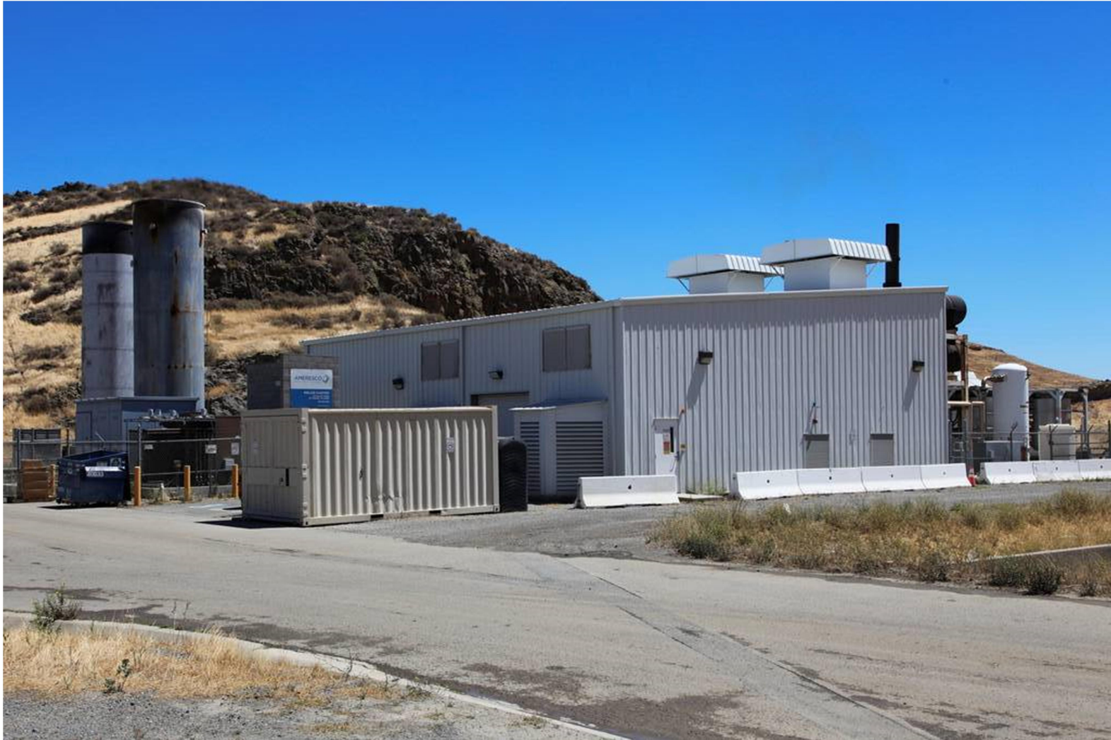
Figure 2 Existing Ameresco LFG Power Plant Looking Northeast
