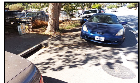
Concrete Sidewalk terminates at tree. Inadequate pedestrian facilities with cars parking on path in Segment 2.
