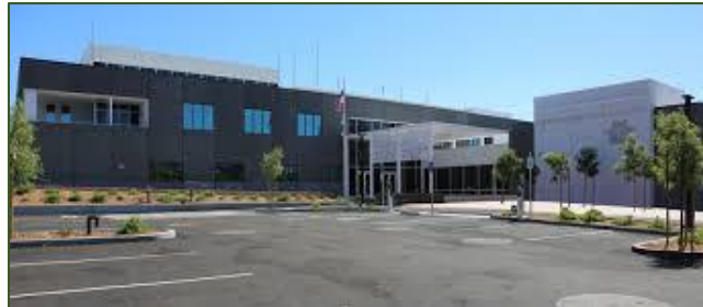
EMERGENCY OPERATIONS CENTER
