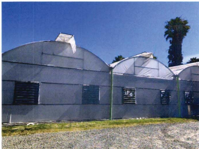
South facing Greenhouse wall with louvered fan windows.
