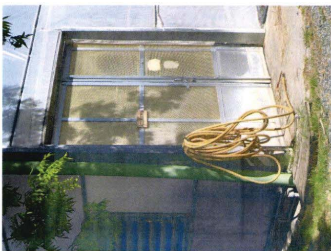
Existing Door Access to Greenhouse
