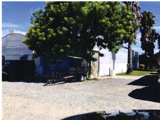
Existing Greenhouse, looking north
