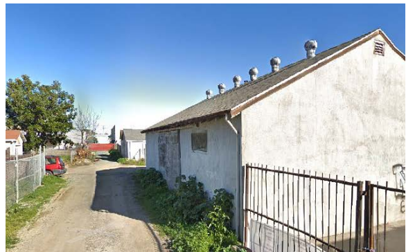
362 Parker Ave _ Office
