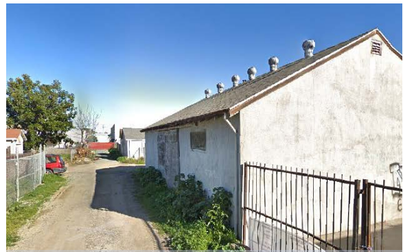
362 Parker Ave _ Office
