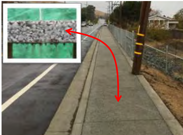
Figure 9: Post-Construction Image with bike lanes and new sidewalk with permeable concrete
