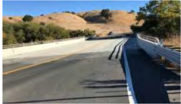
Figure 10: Post Construction Image of Alhambra Valley Road
