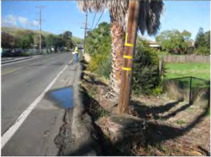
Figure 8: Pre-Construction Image of Pacific Avenue (above)
