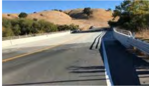
Figure 10: Post Construction Image of Alhambra Valley Road
