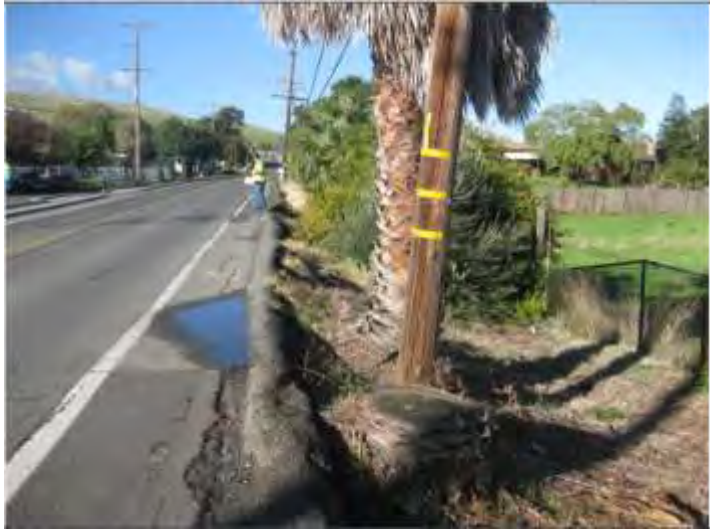
Figure 8: Pre-Construction Image of Pacific Avenue (above)
