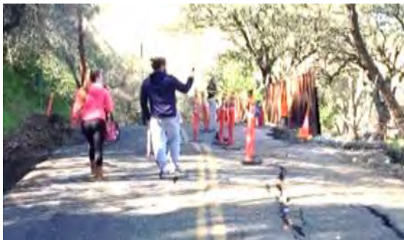
Figure 13: Resident surveying the Morgan Territory Washout in Central County
