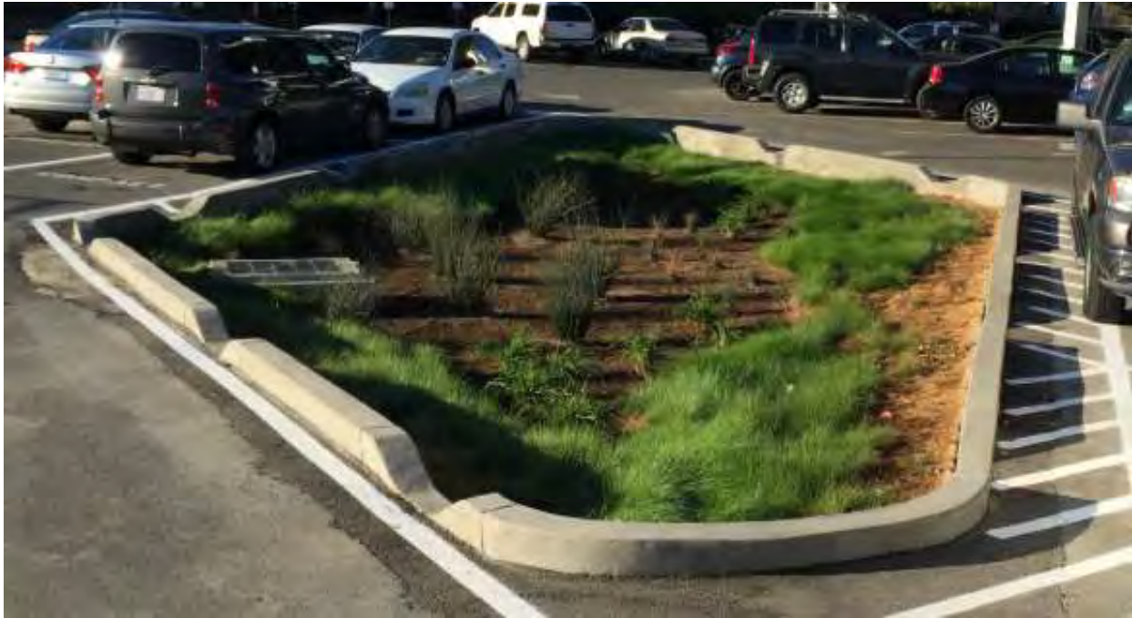
Figure 5: Sample Bioretention Basin Project to support our Green Infrastructure Policy
