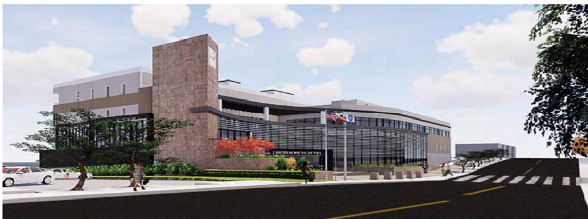
Figure 3 New Admin Building Southwest Corner
