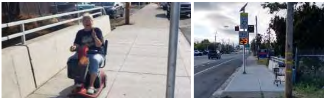
Figure 7: Post-construction image of the new sidewalk/culvert extension
