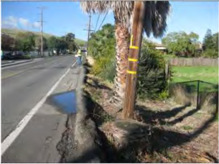
Figure 8: Pre-Construction Image of Pacific Avenue (above)
