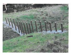
Heavy rain events mobilized off-lite debris into several storm drains, causing blockages and flooding. The Deer Meadow Drive Storm Debris Catemaent Improvement will consist of a series of upstream debris catchments.
