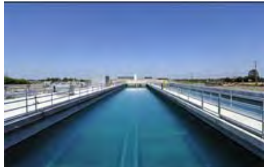
City of Brentwood Water Treatment Plant.
