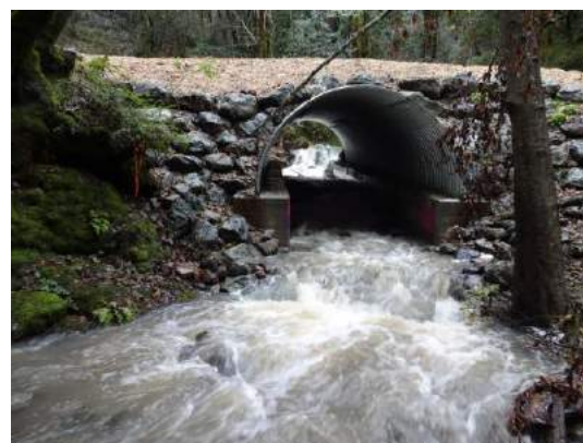
Dog Creek Culvert
