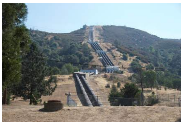
Regional efforts to help increase water supply reliability include regional interties.
