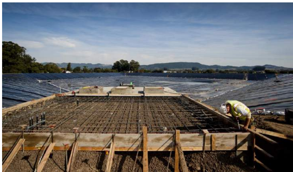
Sonoma Valley Recycled Water Reservoir under Construction
