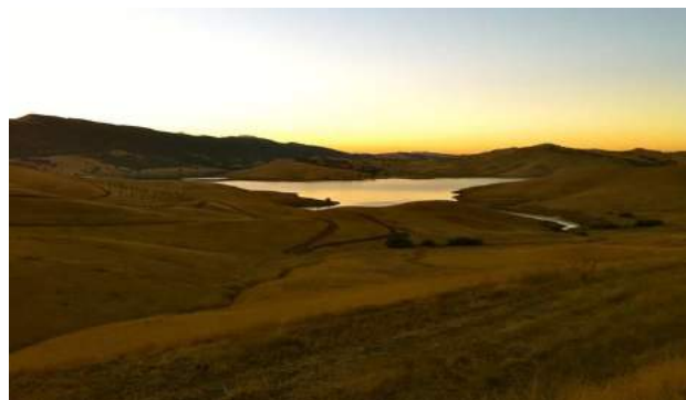
Los Vaqueros Reservoir is an important surface storage reservoir in Contra Costa County.
