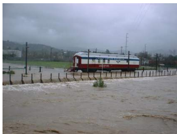
Napa River Flood Control Project
