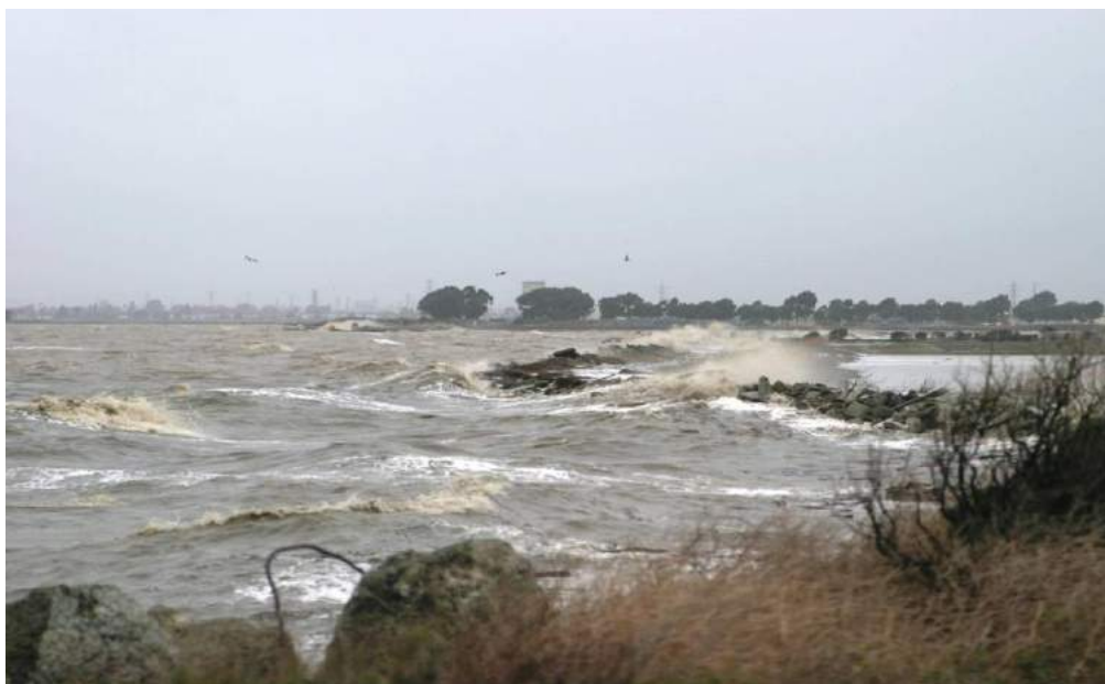
Flooding resulting from sea level rise can threaten shoreline infrastructure.
