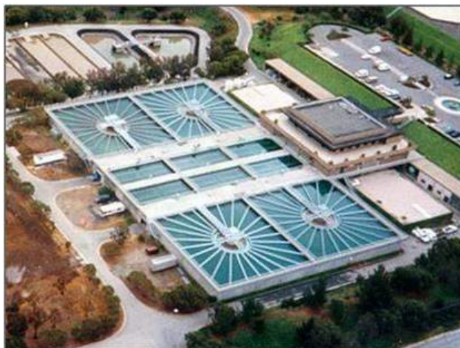
Rinconada Water Treatment Plant, SCVWD
