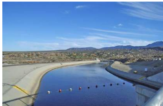
DWR South Bay Aqueduct
