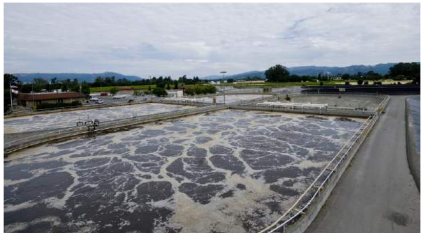
Wastewater treatment plant aeration basin.
