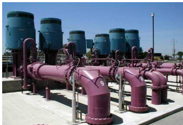
Recycled water is a drought-resistant supply that can contribute to improved supply reliability.
