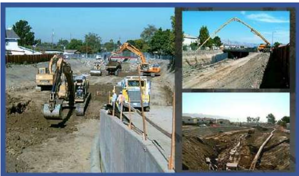
Grant-funded flood protection project, Lower Silver Creek, Santa Clara Co.
