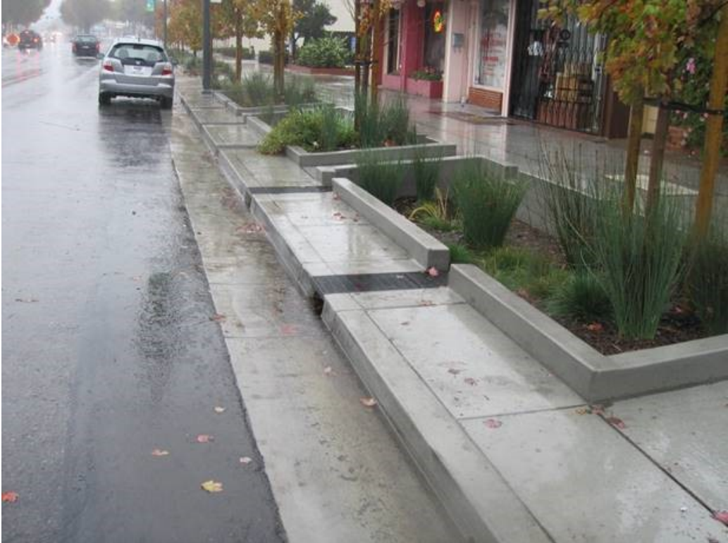
Figure 1: Off-line system in El Cerrito where low flow is diverted to the sidewalk planter and high flows continue down the gutter.
