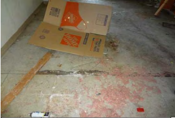
#13 CRACKED INTERIOR SLAB
