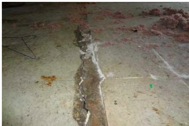
#12 CRACKED INTERIOR SLAB
