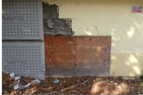
#20 DAMAGED EXTERIOR STUCCO
