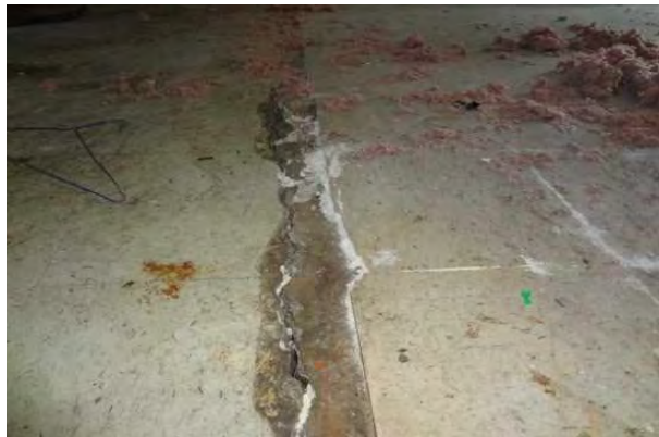
#12 CRACKED INTERIOR SLAB
