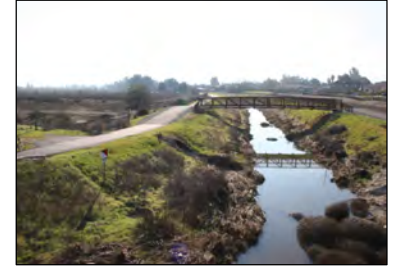
Looking upstream from UPRR tracks
