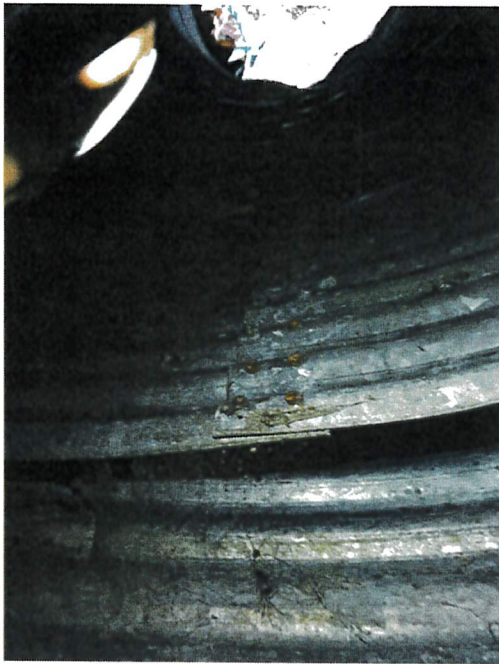
4) Culvert joint repair
