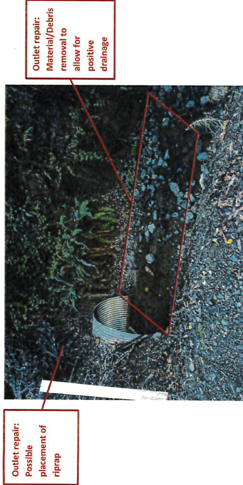
3) Culvert outlet repair
