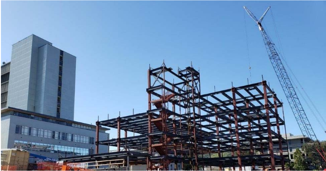
Figure 2 County Administration Building
