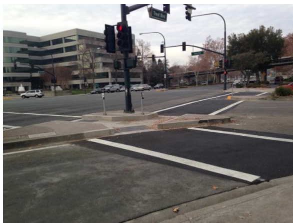
Photo 16 View west on the east side of Oak Road, showing northbound free right turn lane and splitter island: cars speed around the corner, or block the crosswalk while waiting to merge.
