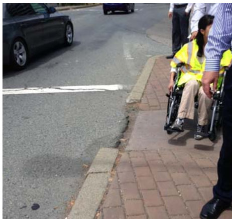
Photo 10 North crosswalk of Buskirk Avenue typifies some of the existing curb ramps with uneven surfaces difficult to traverse for those with mobility impairments.
