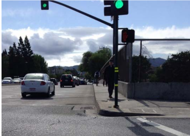
Photo 8 View west of the I-680 overcrossing sidewalk from Buskirk Avenue. Current 5' wide sidewalk is insufficient for two-way pedestrian use. Bicyclists were observed using this facility to travel east and west instead of using the roadway.
