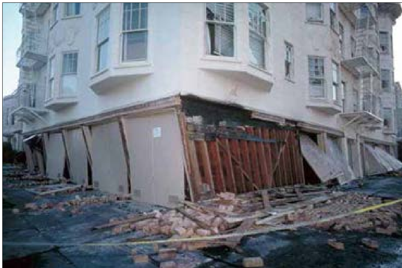
Figure 8-12. Soft-Story Damage from 1989 Loma Prieta Earthquake
